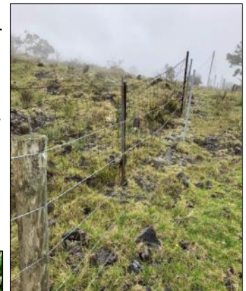
Cross fence using 5 barbed wires on the T-posts. The T-posts are new as well. Note the old fence behind the new fence.
