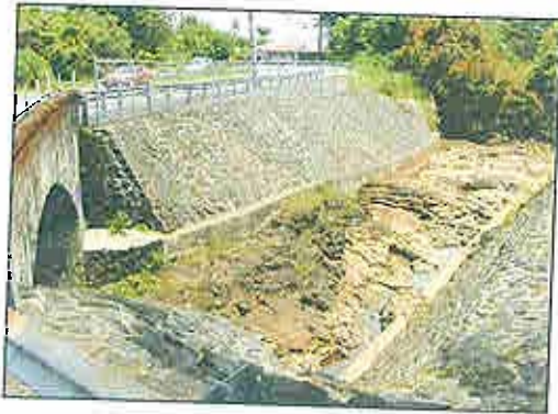
Streambank protection project at the Chong bridge site.
