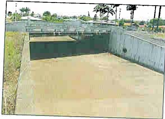
Kawailani bridge and flood control channel project completed in 2005.
