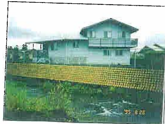
Geotextile Streambank Stabilization and Protection project.
